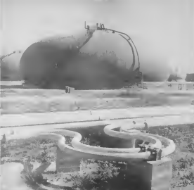
WHAT'S that? Visitors ask if expansion loop in lines. How much will that tank hold? They pour...
